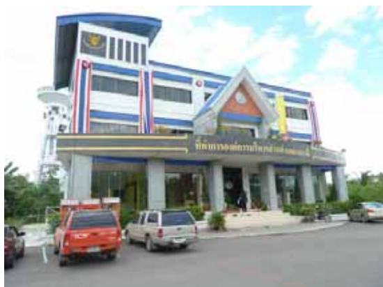
Fig. 3 The Bang-nanglee Sub-District Administrative Office
