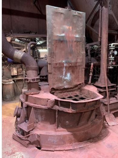
Figure 1. Mixers used for raw materials dispersion in water at ILPEA
