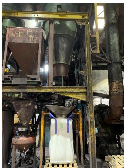
Figure 3. Milling systems at ILPEA
