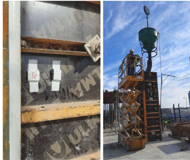
Fig. 19. Collection of formwork accelerations during vibration of columns concrete.
