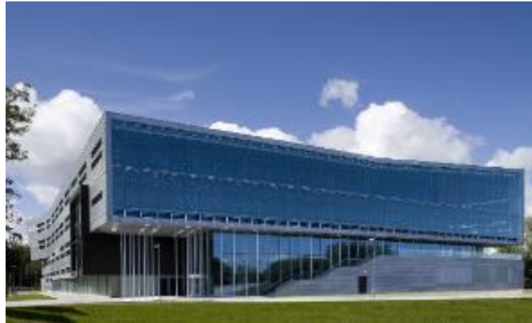
Alice Perry Engineering Building (Galway)
