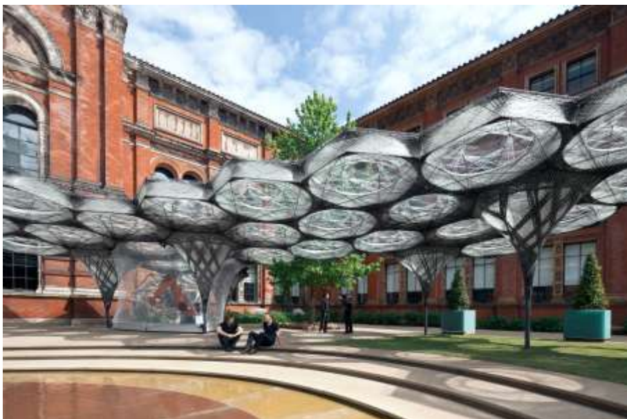
Figure 6 Structural differentiation of fibre layout for columns and roof components (photo: NAARO)
