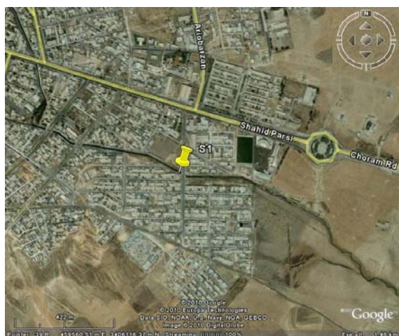
Fig. 4 Station 1 is located on the main waste water collection canal in Dehdasht
