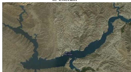
Fig. 7 The Kowsar dam reservoir
