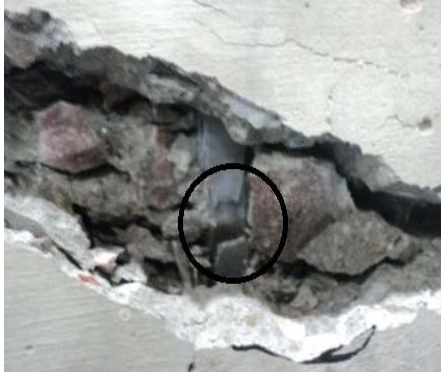
Fig. 5the necking phenomenon of steel strips
