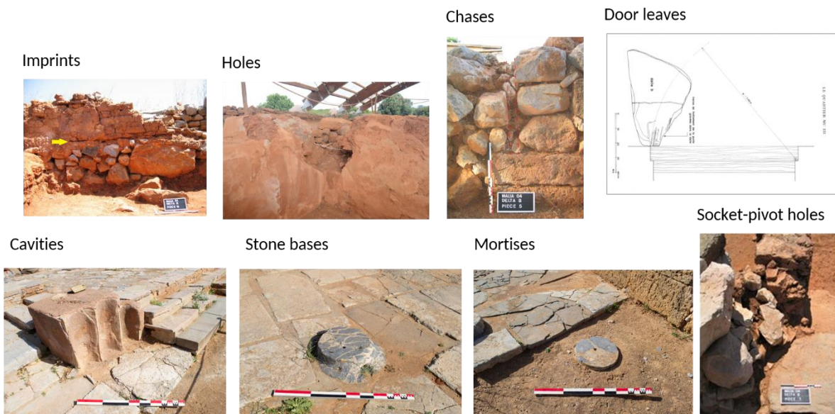
Figure 2 – Indirect evidence for timber use (door leaves' drawing after Poursat, 2005).
