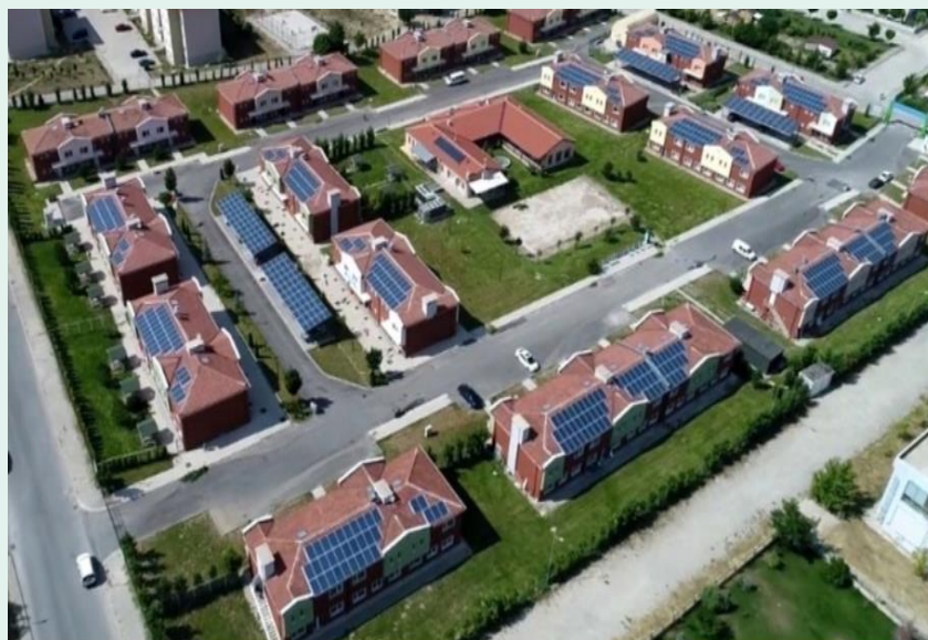
Figure 91: Field 1PV Area
