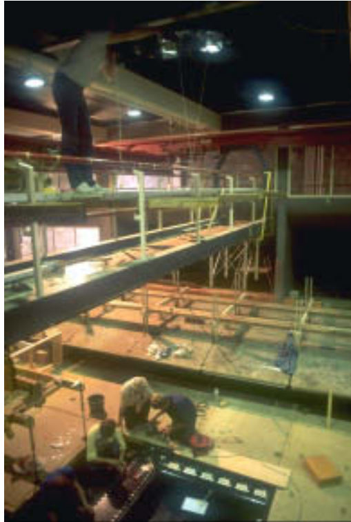
Figure 2: Close to the beach and air-flow return section, the 10 m wide corridor section of the Delft wind wave facility (see Figure 1) opens to a 30 m wide and 5.5 m high end section. Instruments can directly built into the bottom of the facility, replacing 2 \times 2 \text{ m}^2 large and 0.2 m high concrete plates. With a traveling bridge instruments can be mounted at the ceiling. (For color figure, see Plate 15.)
