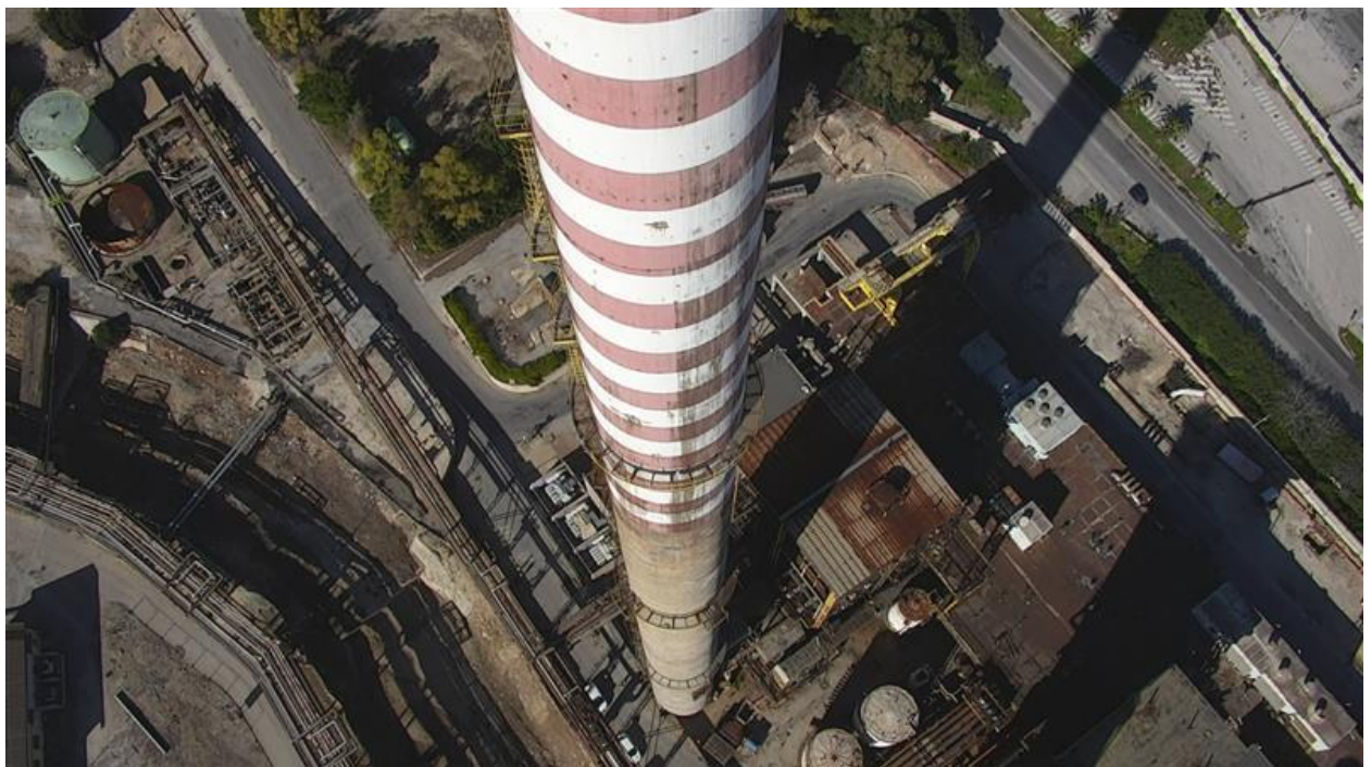
Figure 4 - Example of a visual inspection conducted in a refinery chimney
