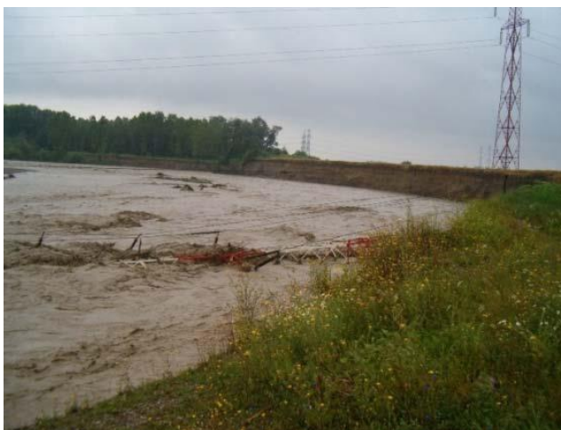
FIGURE 24: 110 KV PYLON COLLAPSE DUE TO RIVERBANK EROSION IN 2005 ROMANIAN FLOOD
