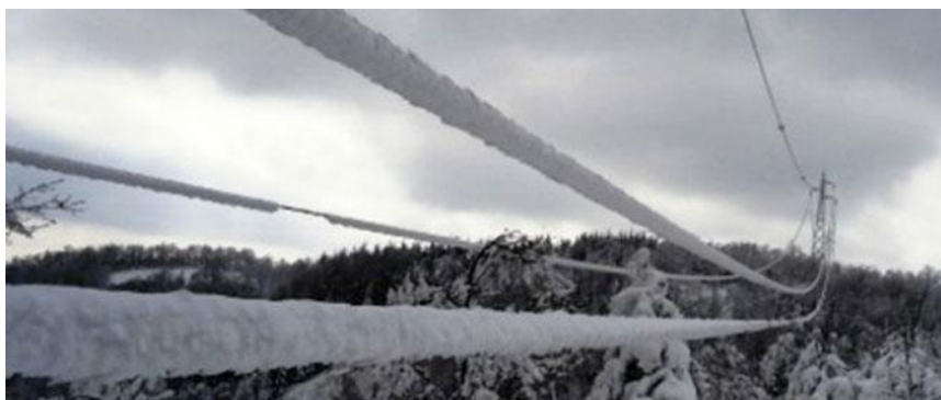
FIGURE 22: CORTINA EVENT WITH ICE SLEEVES ON THE CONDUCTORS
