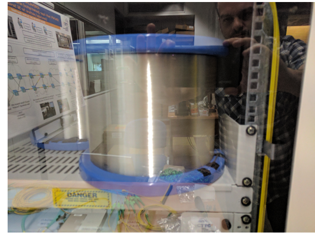
Fig. 5. 35 km of optical fiber in coils.
