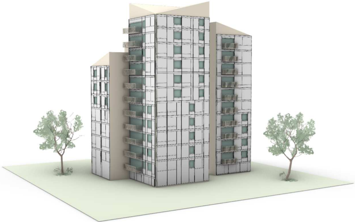
Figure 13. Building model and detailed prefabricated module layout of the demo-building in Milan.
