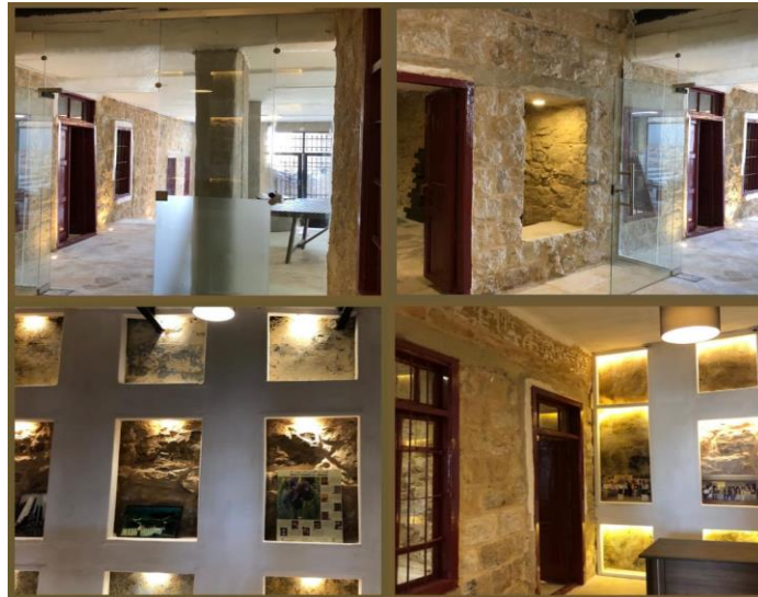
Fig 2: Haddad's heritage house in Jabal Amman after restoration
