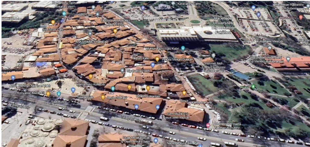
Figure 12. Hamamönü, Altındağ, Ankara (Taken from Google earth)
