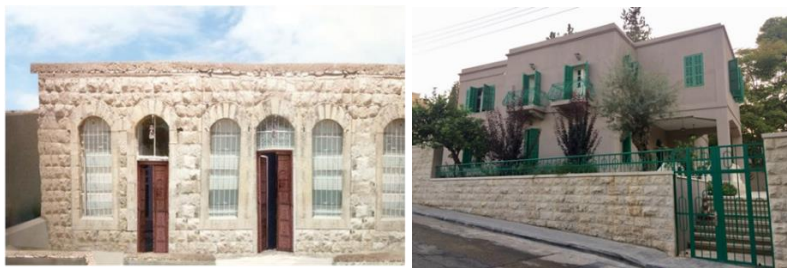
Fig 1 (on the left): Ali Al-Kayed Al-Amayreh House: The first Ottoman-style heritage house in Jabal Al-Hussein. It was built in 1935 from yellow stone to be the first house of this stone on the northern side adjacent to Citadel Mountain in the Jabal Al-Hussein area. (Alghad Newspaper 2015).
