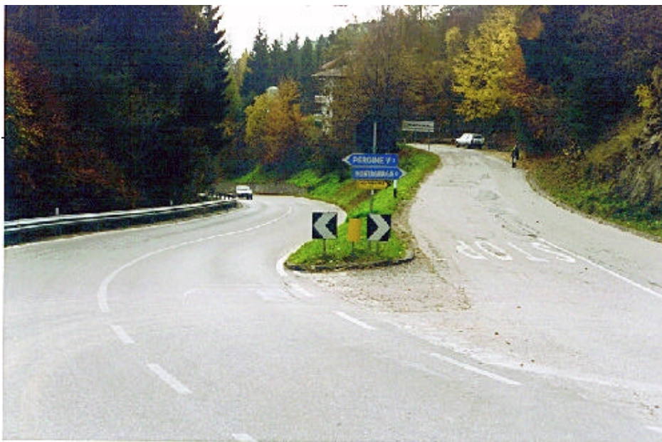
Fig. 6. Montagnaga (Italy). The road on the right is misperceived as running uphill.
