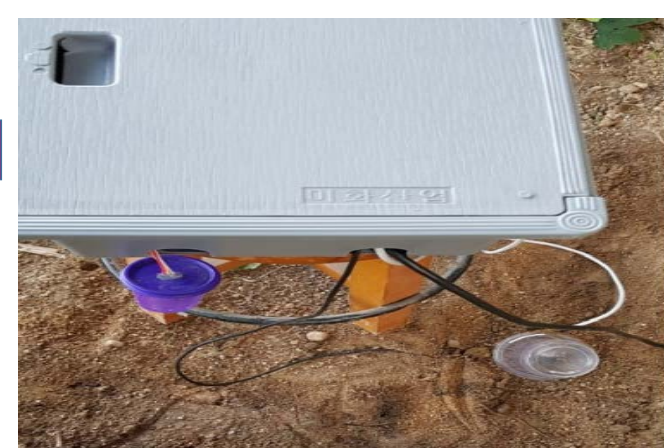
Installation of DAQ on the plum field
