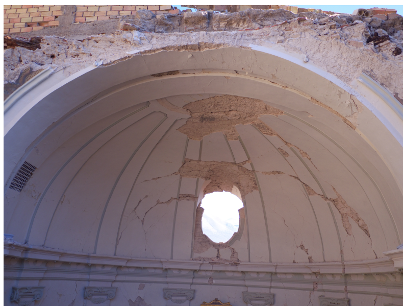
Fig. 5. Norcia – Structural check inside of the dome of the S. Benedetto Church.
