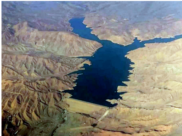
Figure 3. Aerial view of the dam on the "Shirindareh" reservoir (photo: Morteza Behzadfar)
