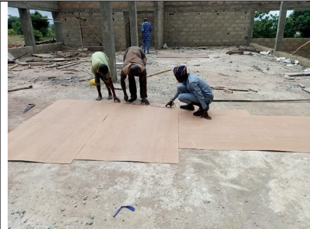
Plate 1: Marking of the segment
