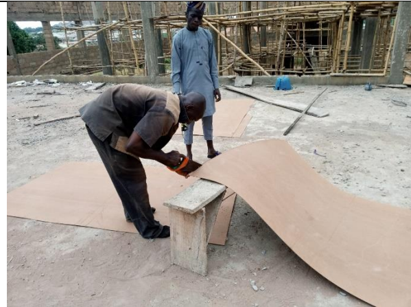
Plate 2: Cutting of the segments to form the sphere
