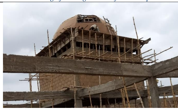
Plate 4: Covering of the semi-circular skeleton with veneer
