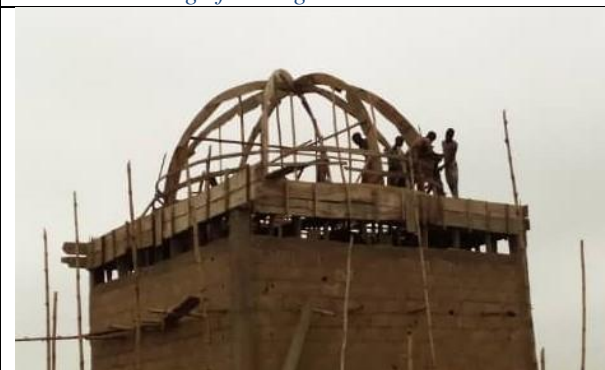
Plate 3: Arrangement of the semi-circular skeleton
