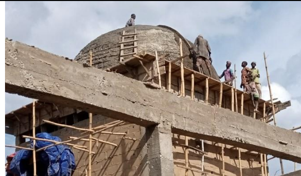
Plate 6: Concrete casting of the dome
