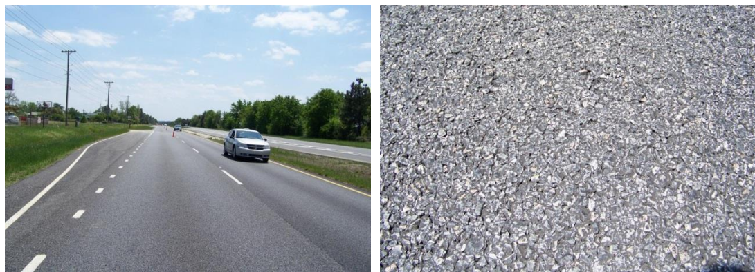
Figure 10-5. Control OGFC surface
