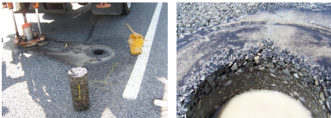
Figure 10-6. Core sample drilling
