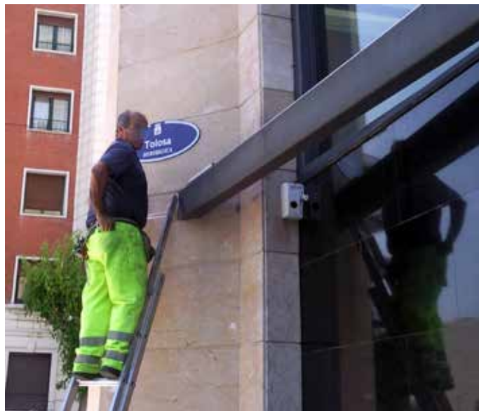
Figure 3.2 Worker putting up a new street sign
