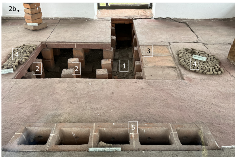
Figure 7 - A reconstruction of a room with hypocaust. Picture from the Jidova, Campulung-Arges. 1-bottom level, 2-pillars made of stalks of bricks, 2b - another possible type of bricks arrangement for sustaining the walking floor, 3-upper layer formed by bricks, 4-“opus signium” - pieces of brick bound with mortar usually placed over #3, 5-double-walls in communication with the double-layer floor with the role in recirculating the heat.
