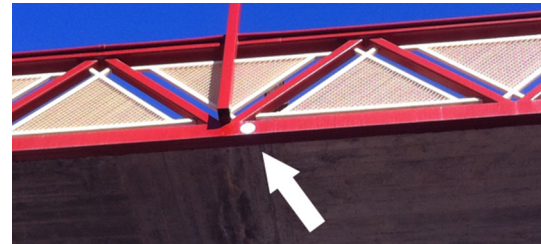
Fig. 2 Detail of the circular white target located in the middle span. A white arrow is pointing the target
