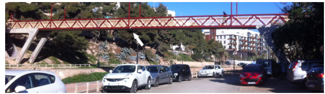
Fig. 1 Footbridge selected for the experiments. A white arrow is showing the target location
