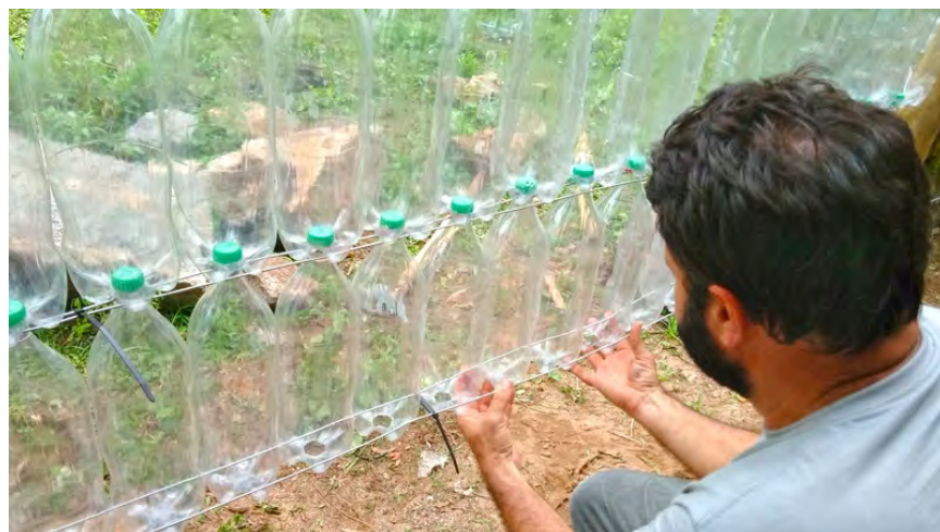
Fig. 11. Construction of the PET Wall in the Botanical Park (courtesy of Ecomuseu Ilha Grande Collection).
