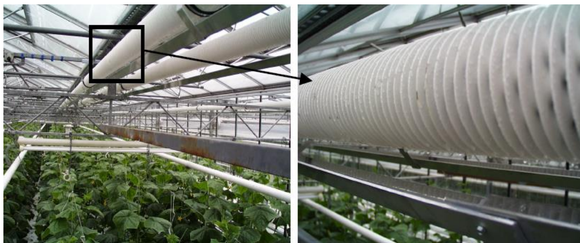
Figure 4. Dehumidification and water recovery system using finned pipes [75].
