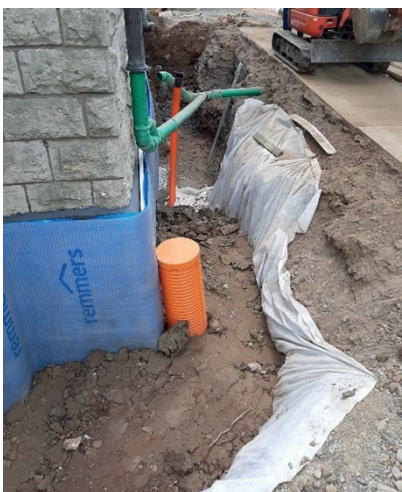
Figure 14: Stabilisation works: filling of the drainage trench, tank installation, perforated pipe for soil moisture management.
