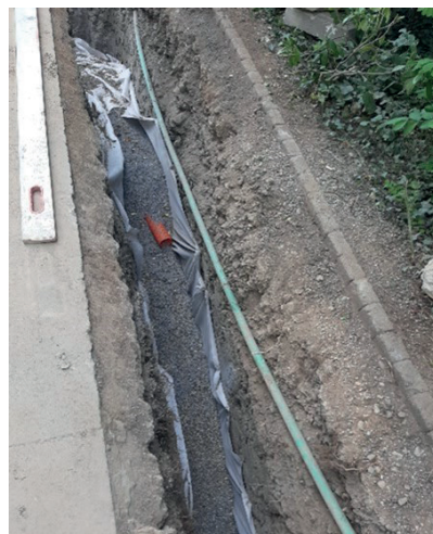
Figure 14: Stabilisation works: filling of the drainage trench, tank installation, perforated pipe for soil moisture management.
