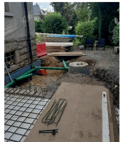
Figure 14: Stabilisation works: filling of the drainage trench, tank installation, perforated pipe for soil moisture management.
