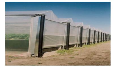
Figure 3.5 Plastic film cladding, used in mild climates Source: *El-Behairy*, 2015.
