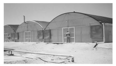
Figure 3.23 A round-arched structure covered with plastic film and permanent shading net, ventilated and cooled by fan and pad system
