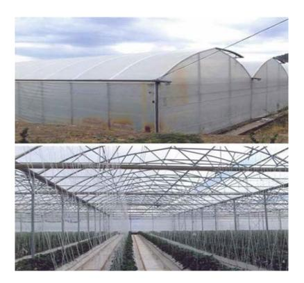
Figure 3.18 Multi-span greenhouse with flap ventilation at the ridge and roll-up ventilation at the sidewall
