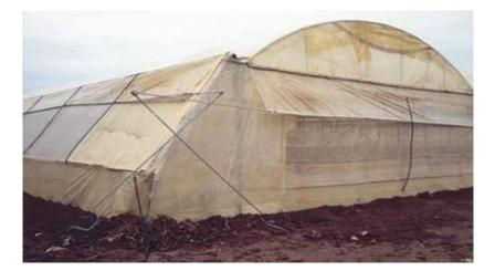
Figure 3.15 Sloped sidewalls covered with insect screens and rolling-up ventilation Source: Von Zabeltitz, 2011. Figure 3.16 shows the possibility of fastening the plastic film by rolling it up on a steel tube. Both the plastic film at the
