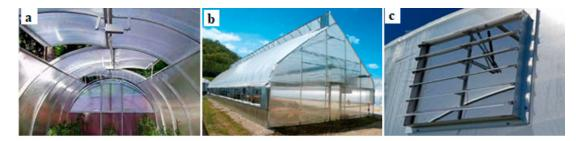
Figure 2. Different types of greenhouse openings: (a) roof vents; (b) ridge vents; (c) side vents.
