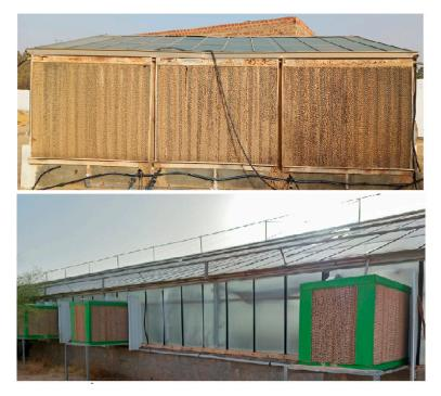
Figure 5. Fan and pad cooling systems for greenhouses at the Institute of Arid Regions (Kebili, Tunisia).
