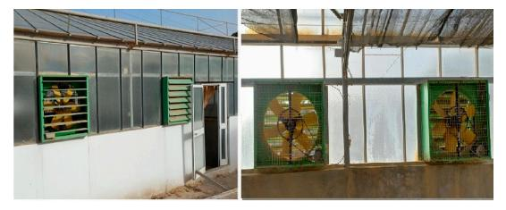
**Figure 3.** A greenhouse equipped with forced ventilation devices at the Institute of Arid Regions (Kebili, Tunisia).
