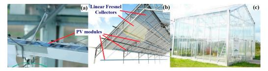
**Figure 10.** (a) The PV modules of the system; (b) the linear Fresnel collectors of the system; (c) the Fresnel greenhouse (The Netherlands). Reprinted with permission from Ref. [103]. Copyright 2011 Elsevier.
