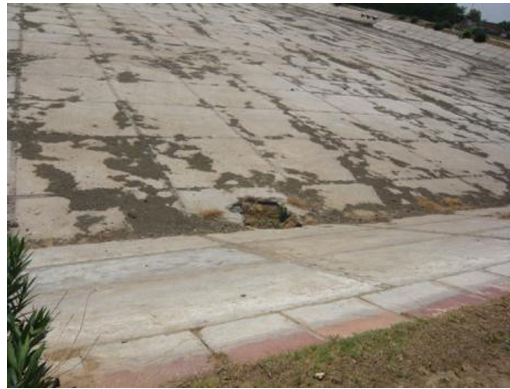
Figure 17.4 Hole in lining of facultative anaerobic pond.
