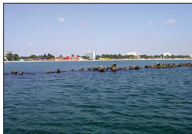
Fig. 7 Breakwater (Mamaia resort)
