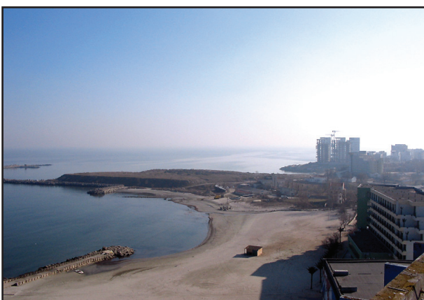
Fig. 6 L- shaped groins, Constanța
