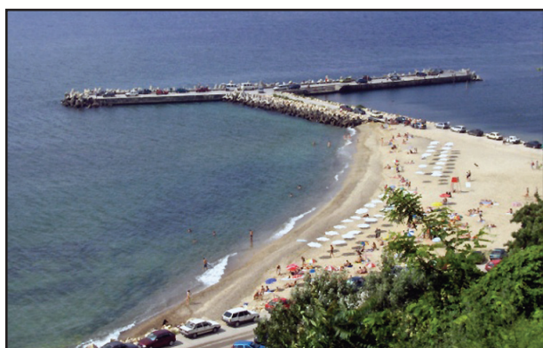
Fig. 2 “Groyne” with port and coast-protection functions
