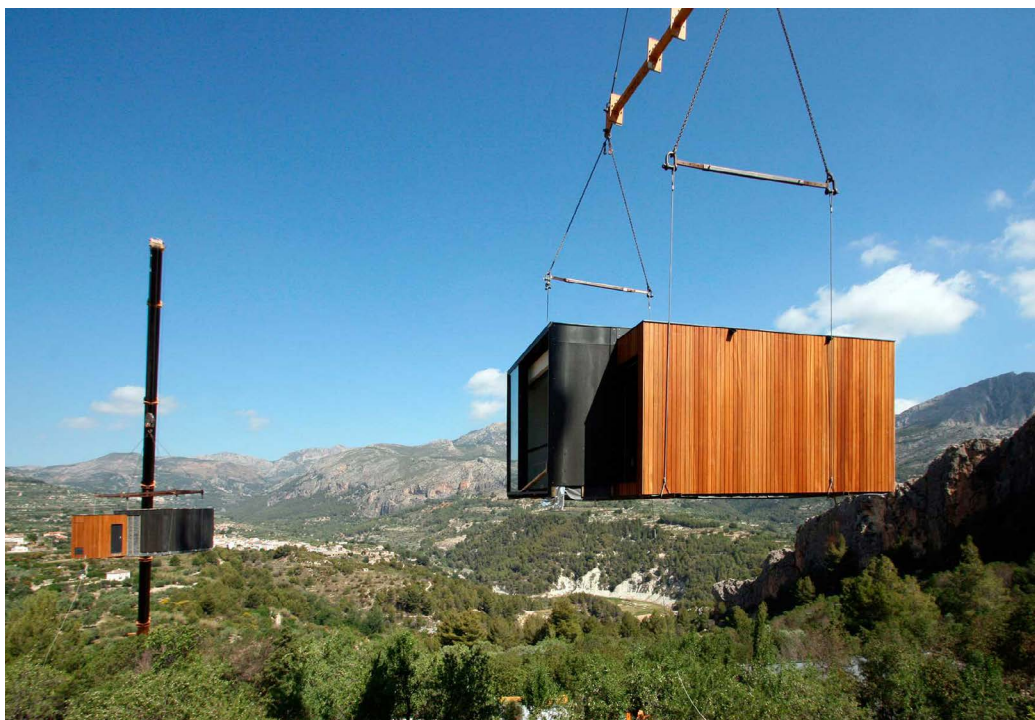
Fig. 3 / Prefabricated modules arriving to site in Vivood hotel. Source: http://vivood.com (2020)
