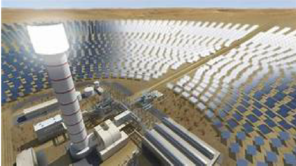
Figure (37) Thermal solar electric power plant using plan mirrors system and a boiler
