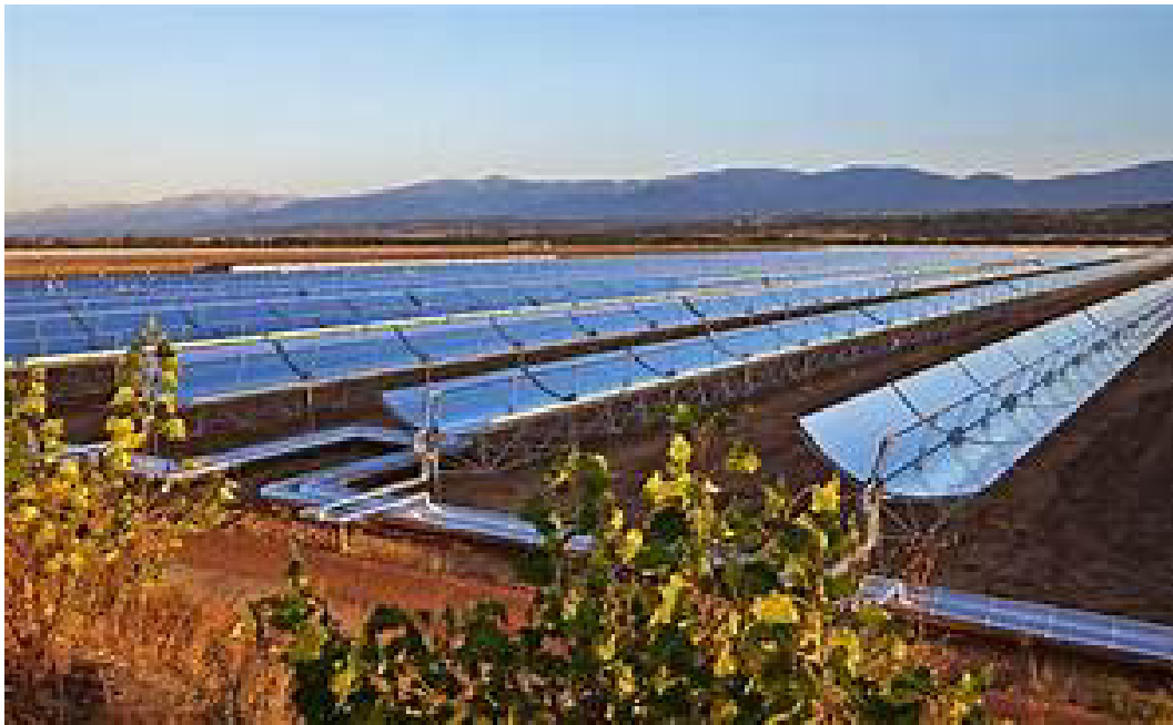
Figure (38) solar electric power plant using cylindrical concave mirror and axial steam pipe.
