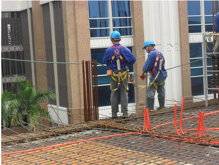
Figure 10: Fall Protection System
