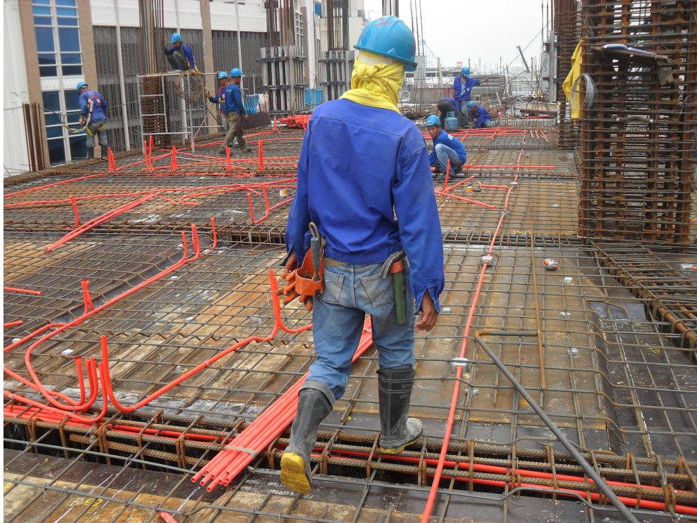
Figure 18: Keeping all tools in place
