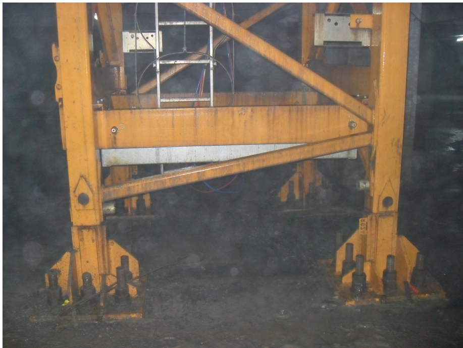
Figure 11: Tower Crane Foundation
