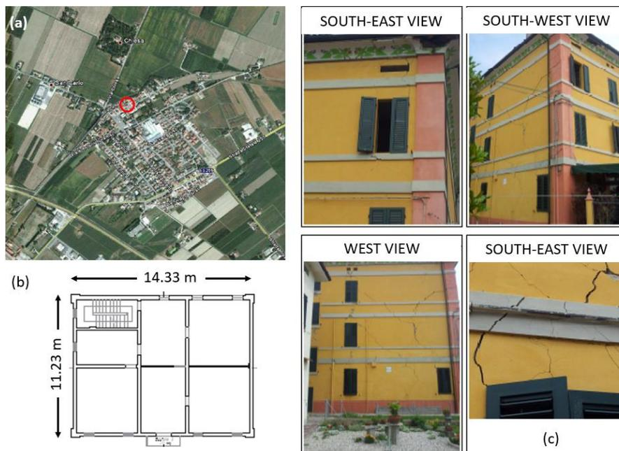
Figure 4. Location of the site (a), plan view of the selected shallow-founded building (b) and observed damage pattern (c).
