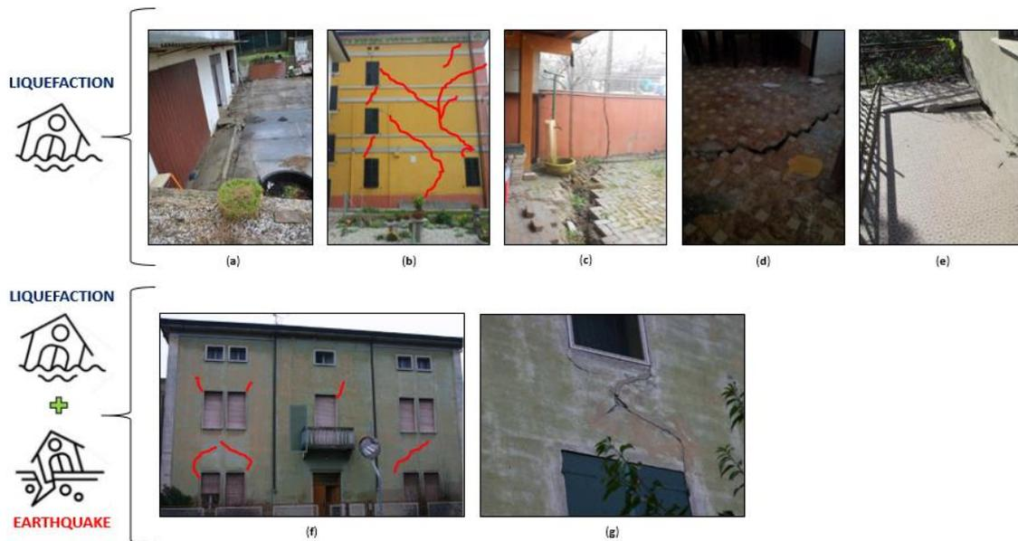
Figure 1. Damage induced by liquefaction.
