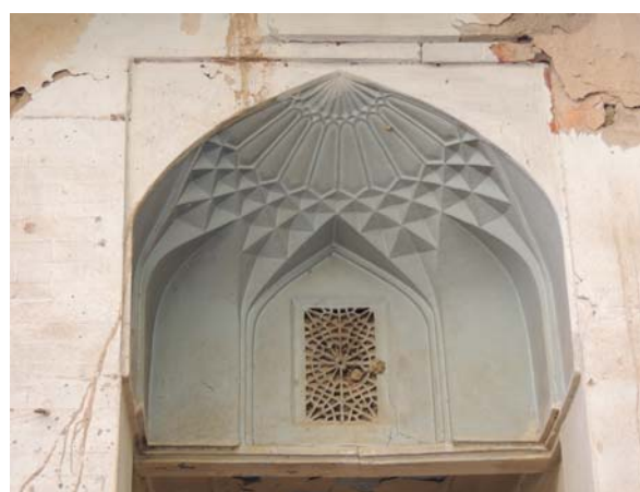
Fig. 4 Façade of Karbandi of Iwan
