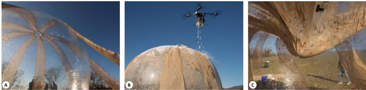
Figure 2: Tests made on pneumatic formwork (from [2]) - A) installation of pneumatic formwork B) matter deposition C) deformation under matter weight and deposition pressure
