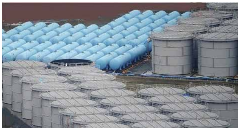
Figure 4. Fraction of tanks with >300,000 m 3 contaminated water at Fukushima power plant.
