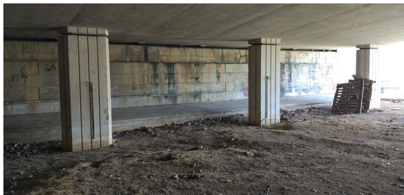
Fig. 8. Photo under the bridge used for mapping.
