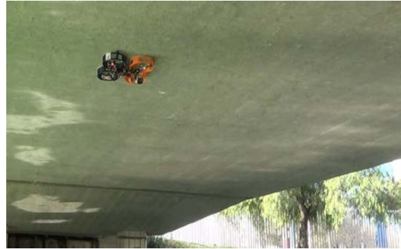
Fig. 1. Multirotor operating in contact with the ceiling.
