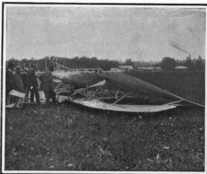
Lefebvre's machine after the accident.
