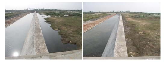
Fig. 9. Photographs of Periyapalayam check dam with and without water (Photo: Kolja Bosch)
