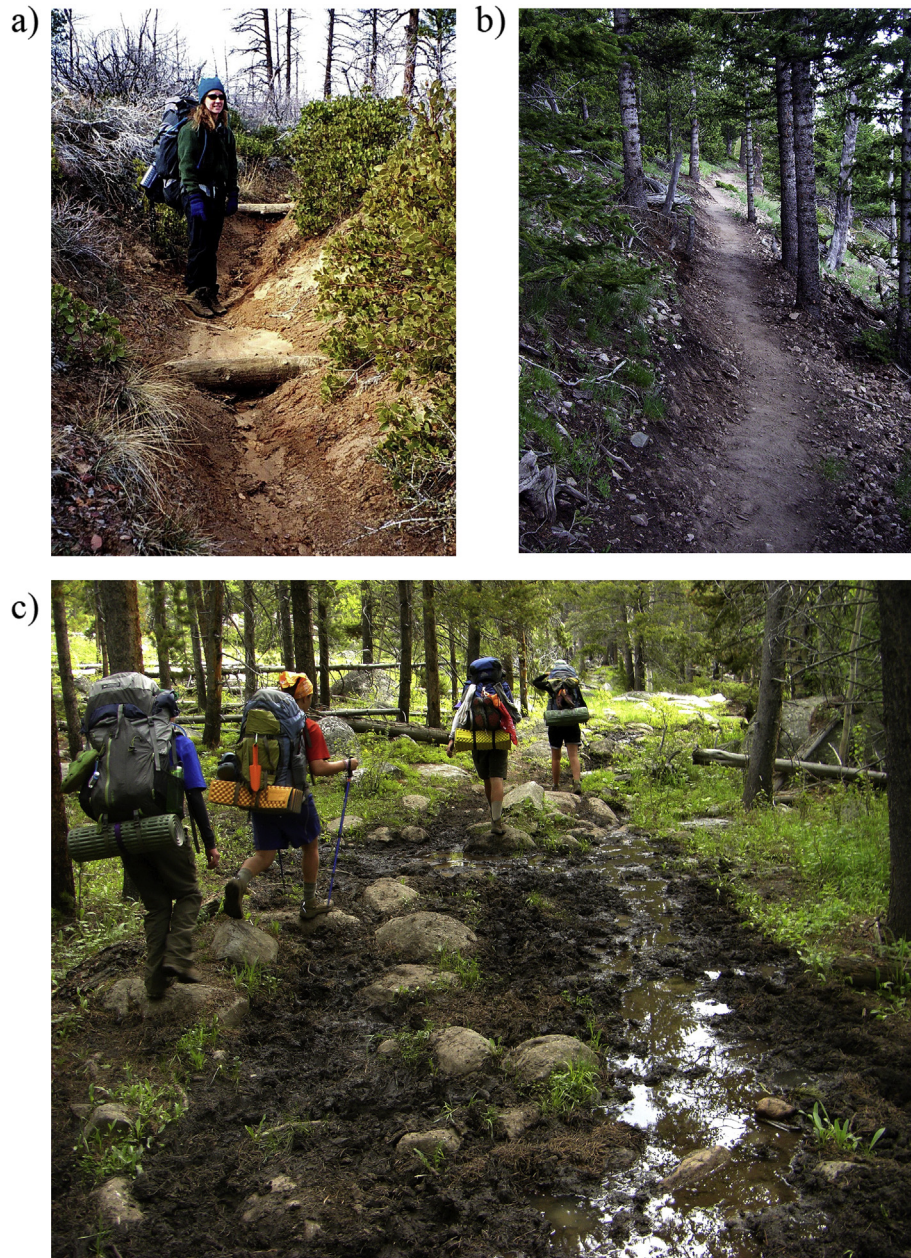
Fig. 2. a) Steep fall-line trails (TSA <22°) erode rapidly. b) Side-hill contour-aligned trails (TSA >69°) resist widening, muddiness, and soil loss. c) TSA is less influential in flat terrain where trail widening and muddiness are common problems. Photos by Jeff Marion.
