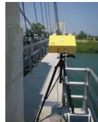
Figure 3. Ibis-S system installed close to the masonry pier to measure the displacements of stays and suspension cables of the Amposta bridge. (after Gentile et al. 2014).
