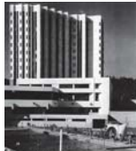
Figure 6. Photo of the measured building (After Negulescu et al. 2013).
