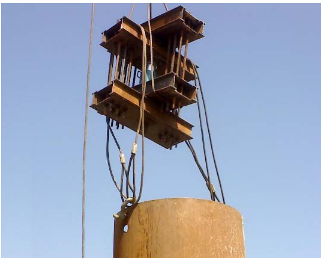
Fig. 3 Imposing tension force to pile
