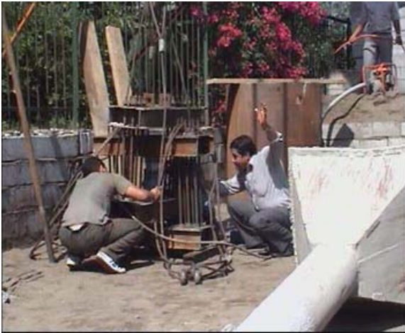
Fig. 2 Hydraulic Jack installation in the frame.
