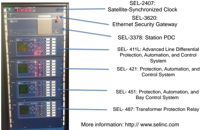
Fig. 4: Phasor Measurement Unit Rack – Four PMUs.
