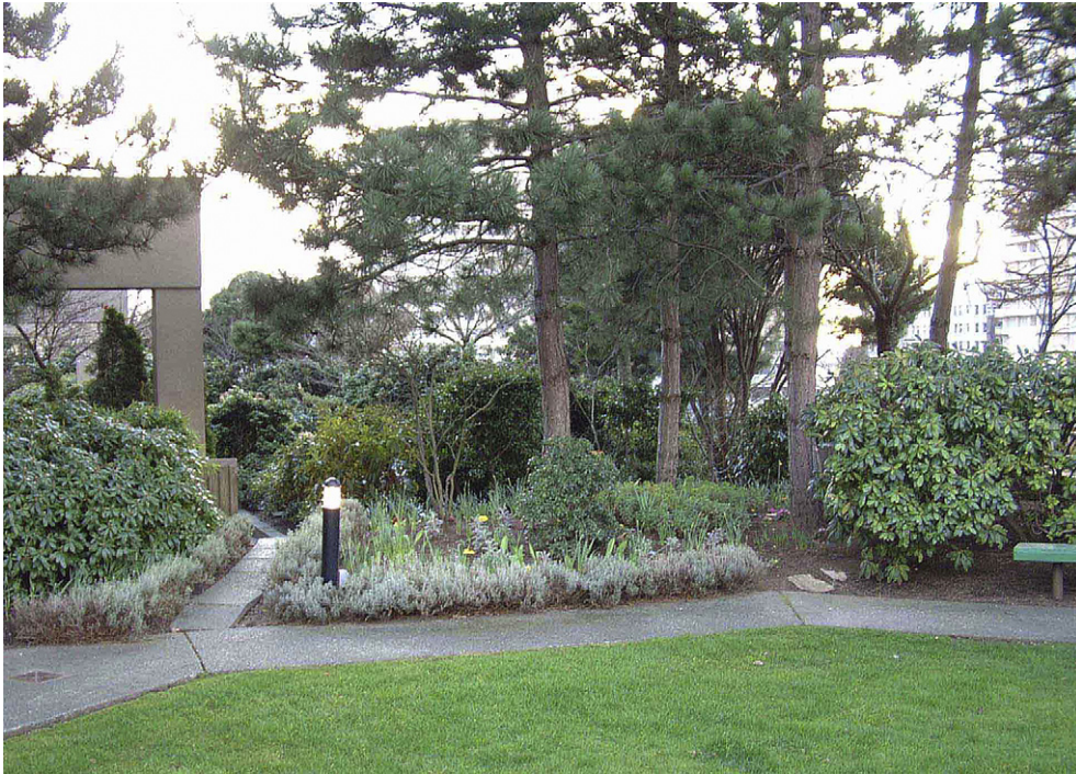
Fig. 1. An intensive green roof on the Coast Plaza Hotel in Vancouver, British Columbia (Photo by Brad Rowe).
