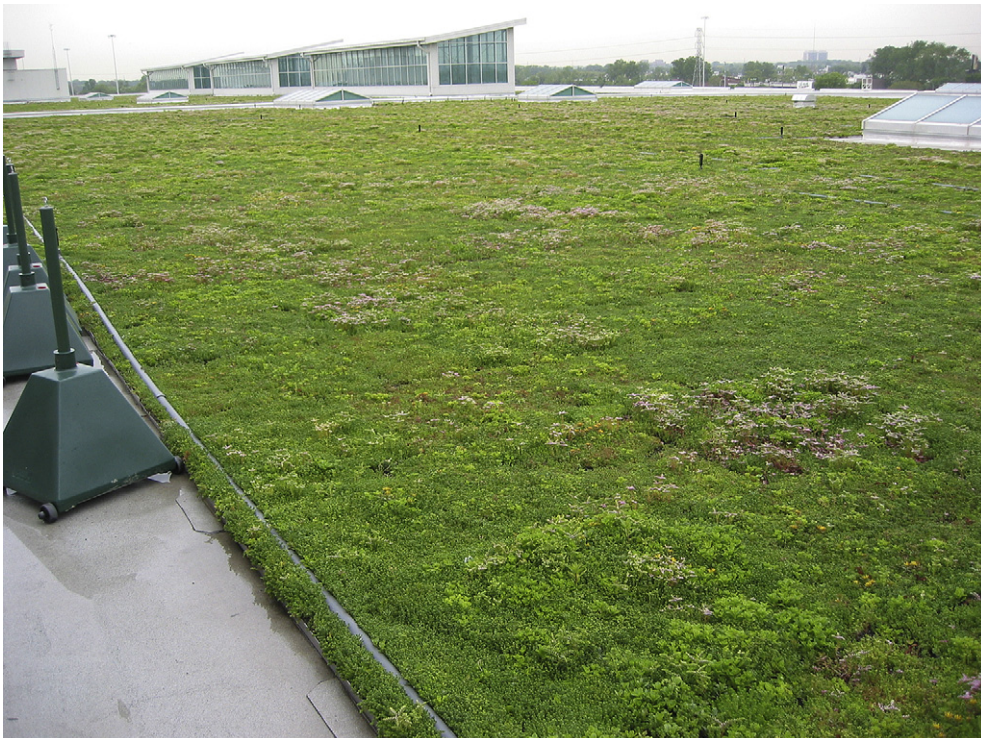
Fig. 2. Portion of a 10.4-acre extensive green roof on an assembly plant at Ford Motor Company in Dearborn, Michigan. Plant material consists of 13 species and cultivars of Sedum (Photo by Brad Rowe).
