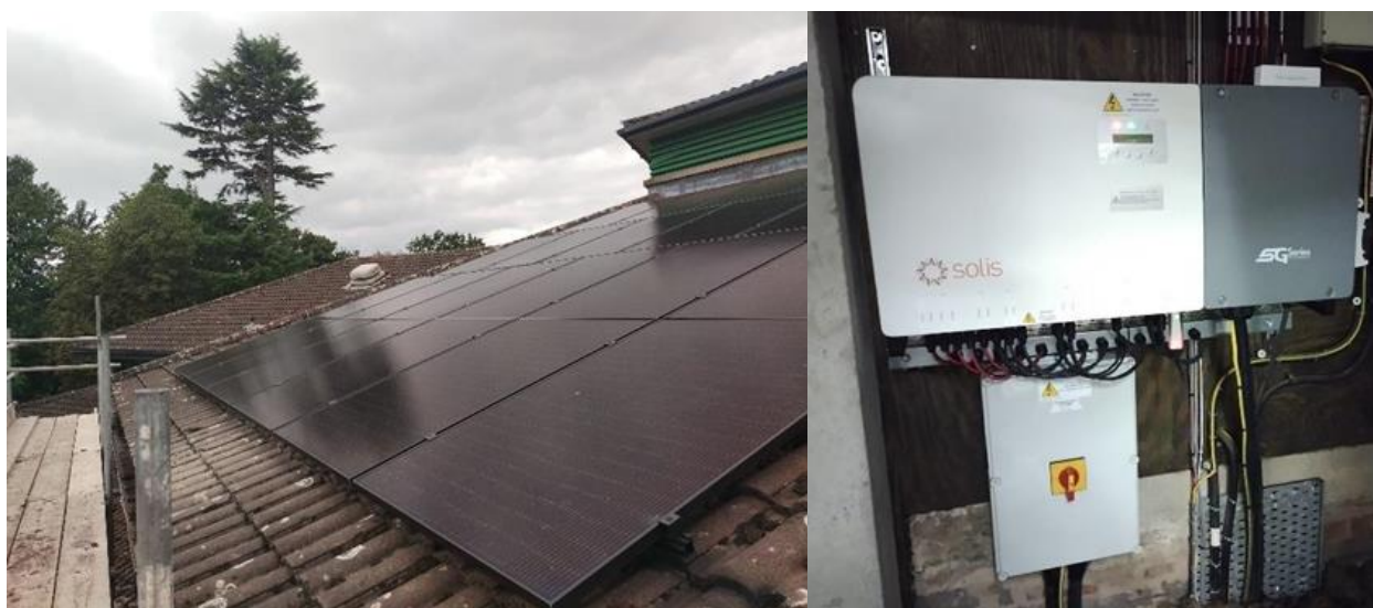
Figure 25 – PV system already installed.
