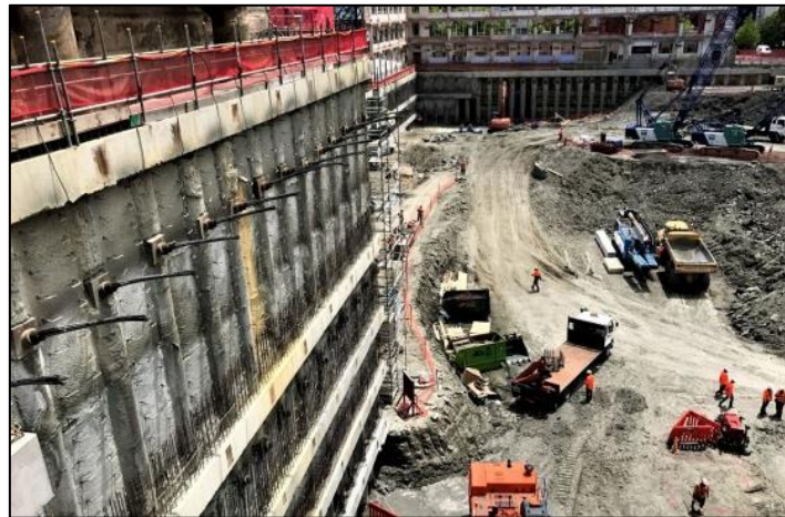
Figure 2.8: Deep excavation during the construction of the New Zealand International Convention Centre (Grouting Services, 2017)
