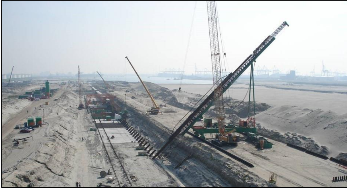
Figure 4.13: Landside picture of the quay wall. The installation of the MV piles is shown in the foreground, with casting of the individual superstructure segments occurring in the background
