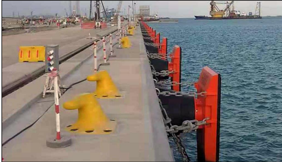
Figure 4.19: Example of fenders (in orange/red) and bollards (in yellow) at a quay wall (Shibata Fender Team, 2016)
